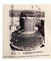
A view of Vermont Yankee Nuclear Power Plant in 1969 shows construction of the drywell.
